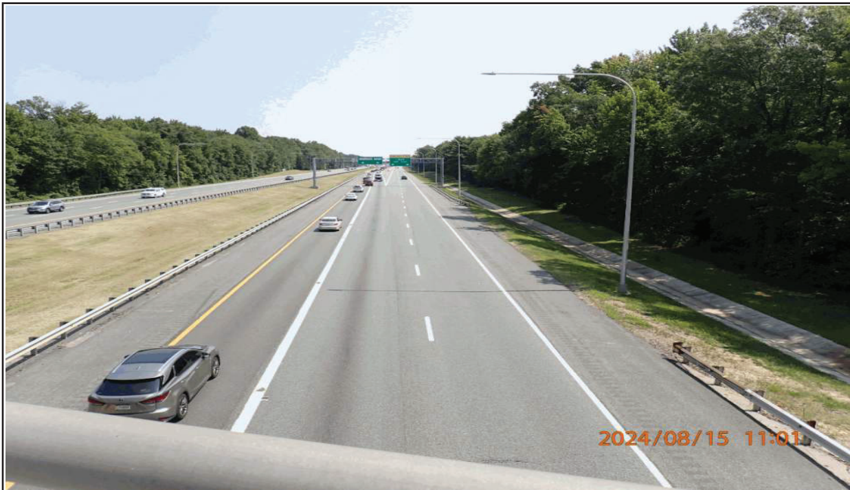
4 UNDER RECORD (SPAN 2 OVER I-95 NB), LOOKING EAST
