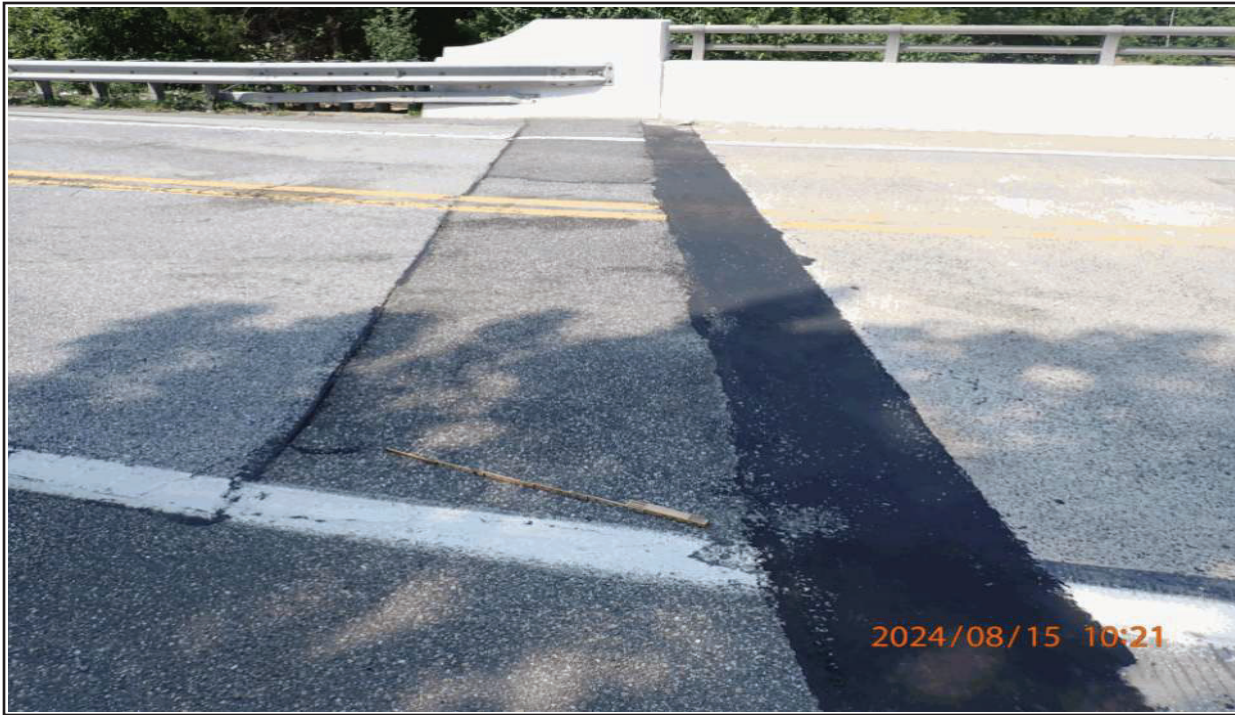
9 SPAN 1 WEARING SURFACE, SOUTH ABUTMENT, SOUTHBOUND LANE - REPAIRED (NOTICE SOUTHEAST APPROACH ROADWAY AT DECK REPAIRED)
