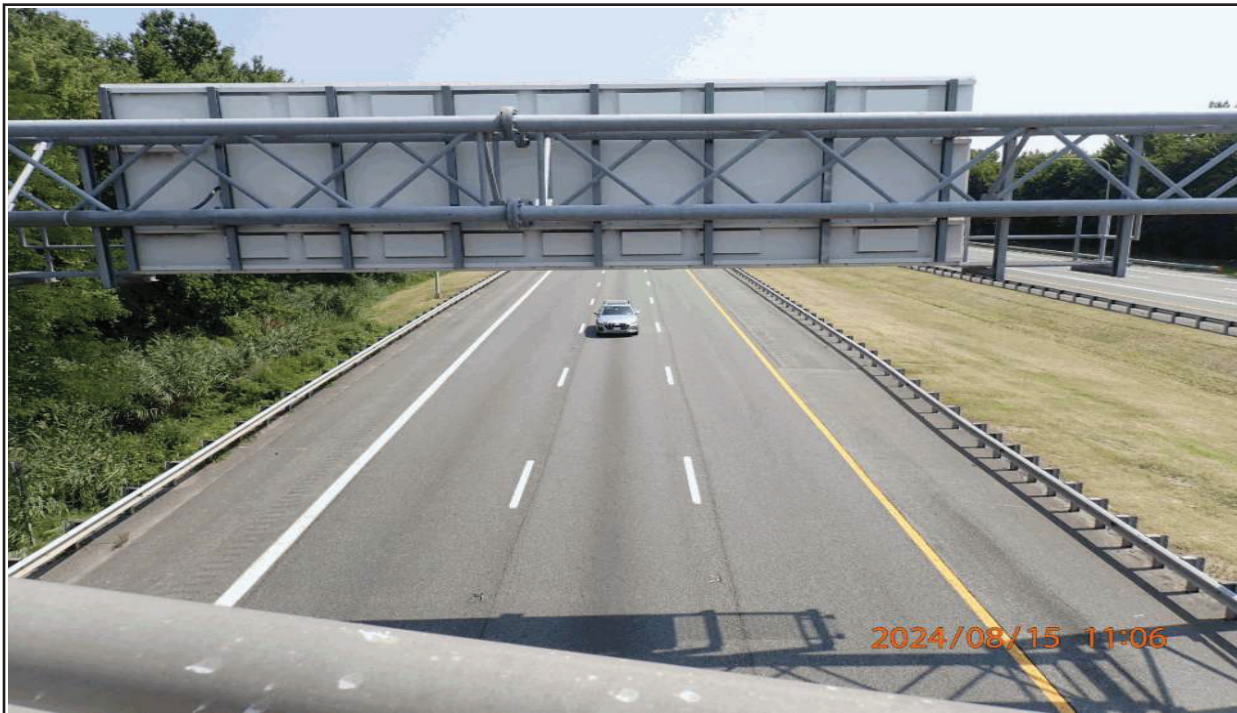
6 UNDER RECORD (SPAN 4 OVER I-95 SB), LOOKING EAST
