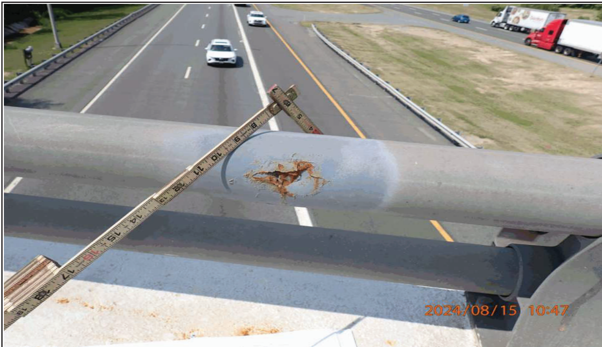
12 SPAN 2 WEST METAL RAIL, TOP HORIZONTAL RAIL - HOLE REPAIRED
