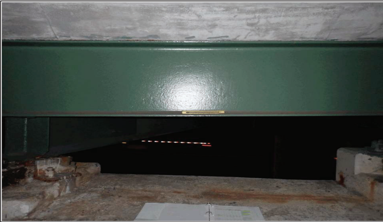
27 SPAN 3, PIER 3, BAY 4 END DIAPHRAGM - TYPICAL PAINT
