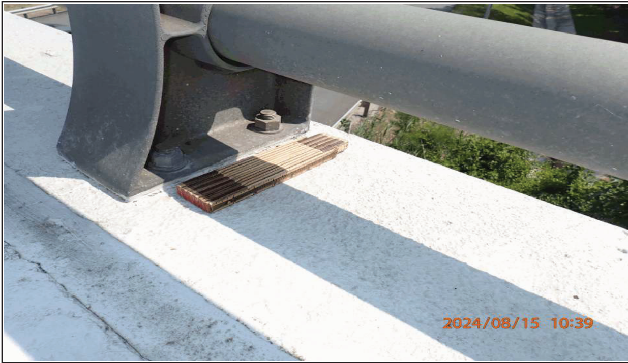
11 SPAN 1, EAST METAL RAIL AT POST 5 - NEW ANCHOR BOLT NUTS
