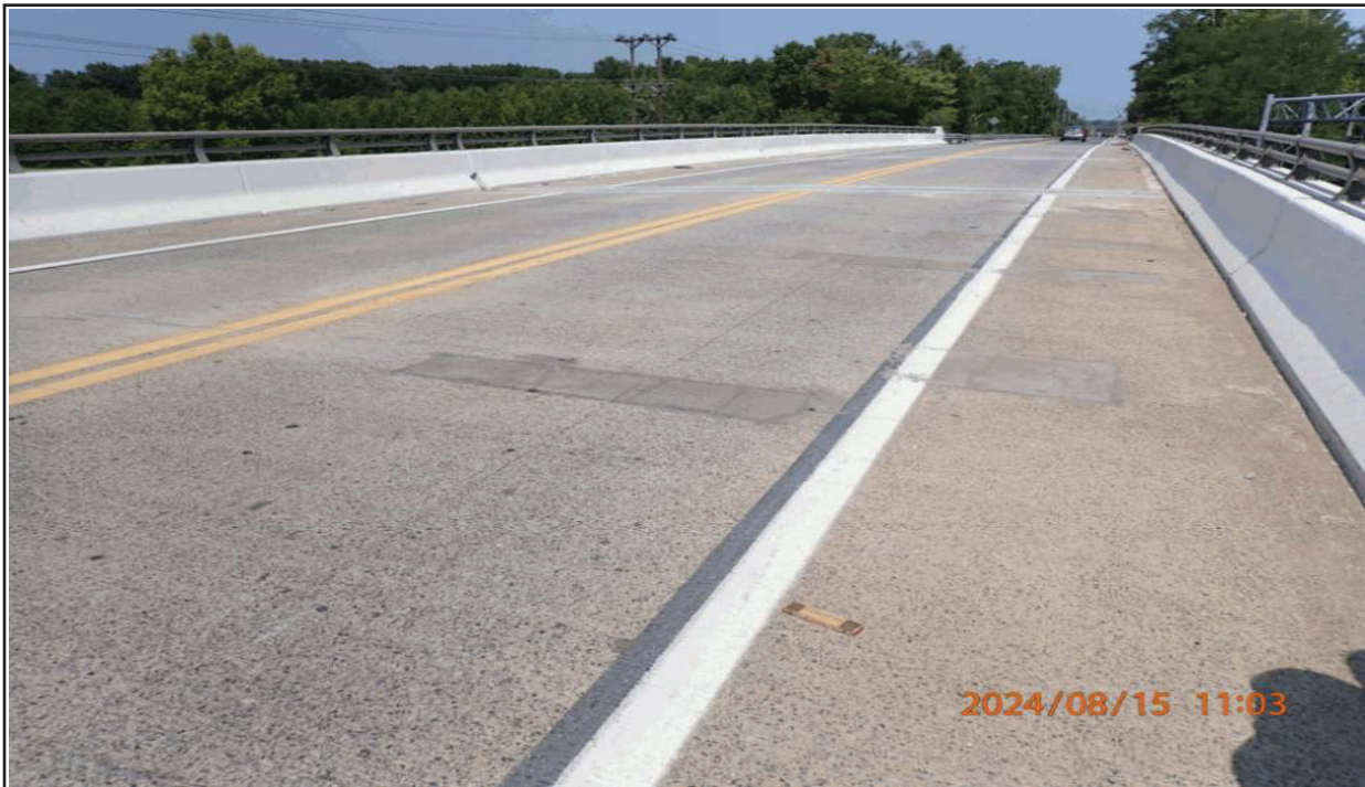
8 GENERAL VIEW OF WEARING SURFACE (SPAN 2), LOOKING NORTH
