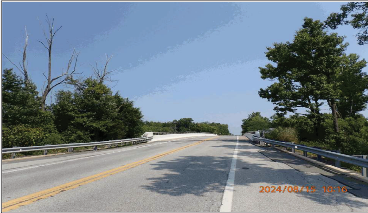
1 SOUTH APPROACH, LOOKING NORTH
