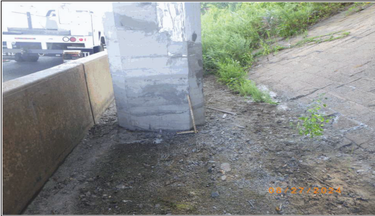
43 SPAN 1, PIER 1, COLUMN 2, WEST FACE - REPAIRED
