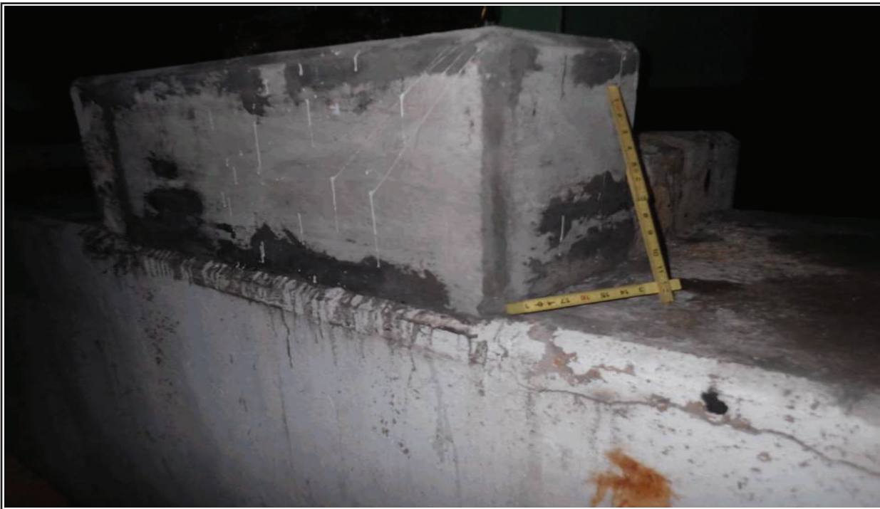
40 PIER 3, SPAN 3, PEDESTAL 3, SOUTH FACE - REPAIRED
