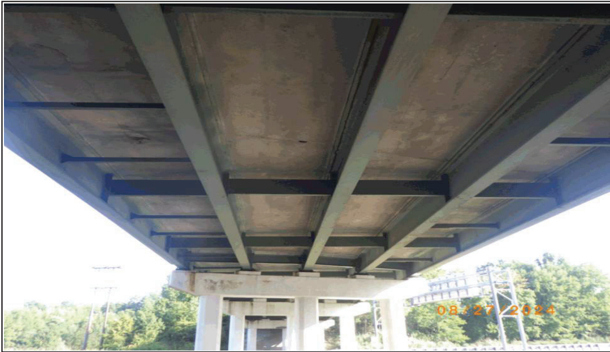
3 GENERAL SUPERSTRUCTURE (SPAN 2), LOOKING NORTH
