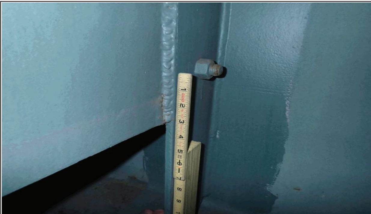
26 SPAN 4, BAY 4, GIRDER 5 AT INTERIOR DIAPHRAGM 1 - EAST VERTICAL WELD CRACK AT BOTTOM
