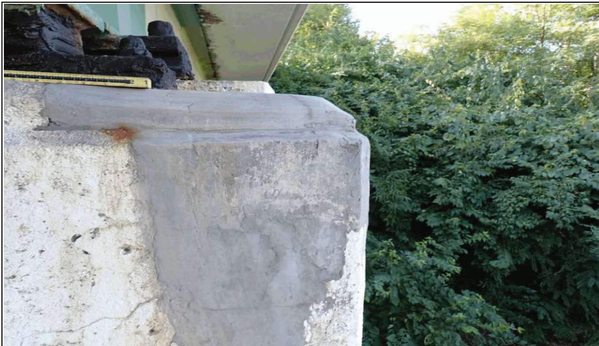
36 PIER 1, PEDESTAL 1 NORTH FACE AND WEST END OF CAP - REPAIRED
