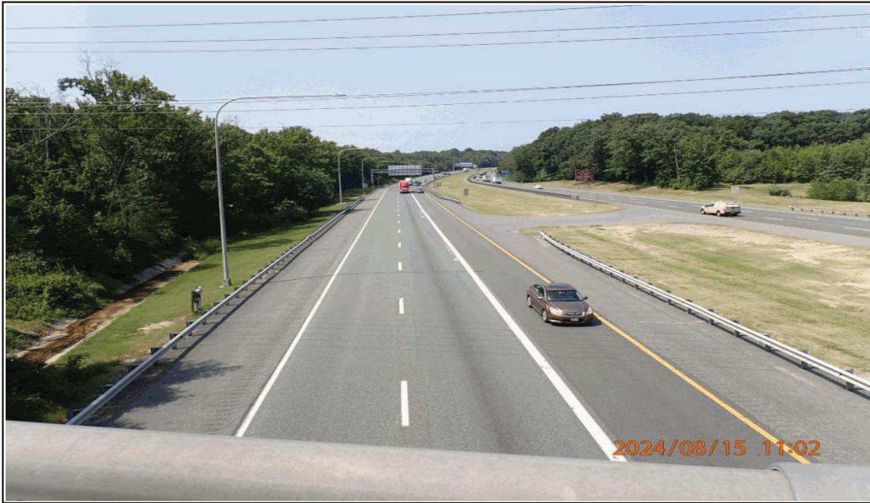
5 UNDER RECORD (SPAN 2 OVER I-95 NB), LOOKING WEST
