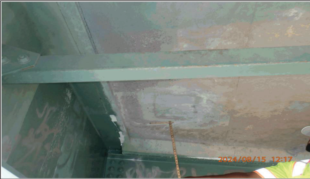
17 SOFFIT, SPAN 5 ADJACENT TO GIRDER 1 - REPAIRED
