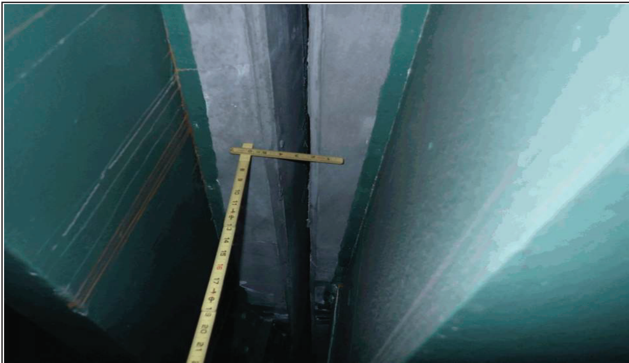
16 SPAN 3, PIER 3, BAY 2 - TYPICAL SOFFIT HAUNCH OVER PIER REPAIR
