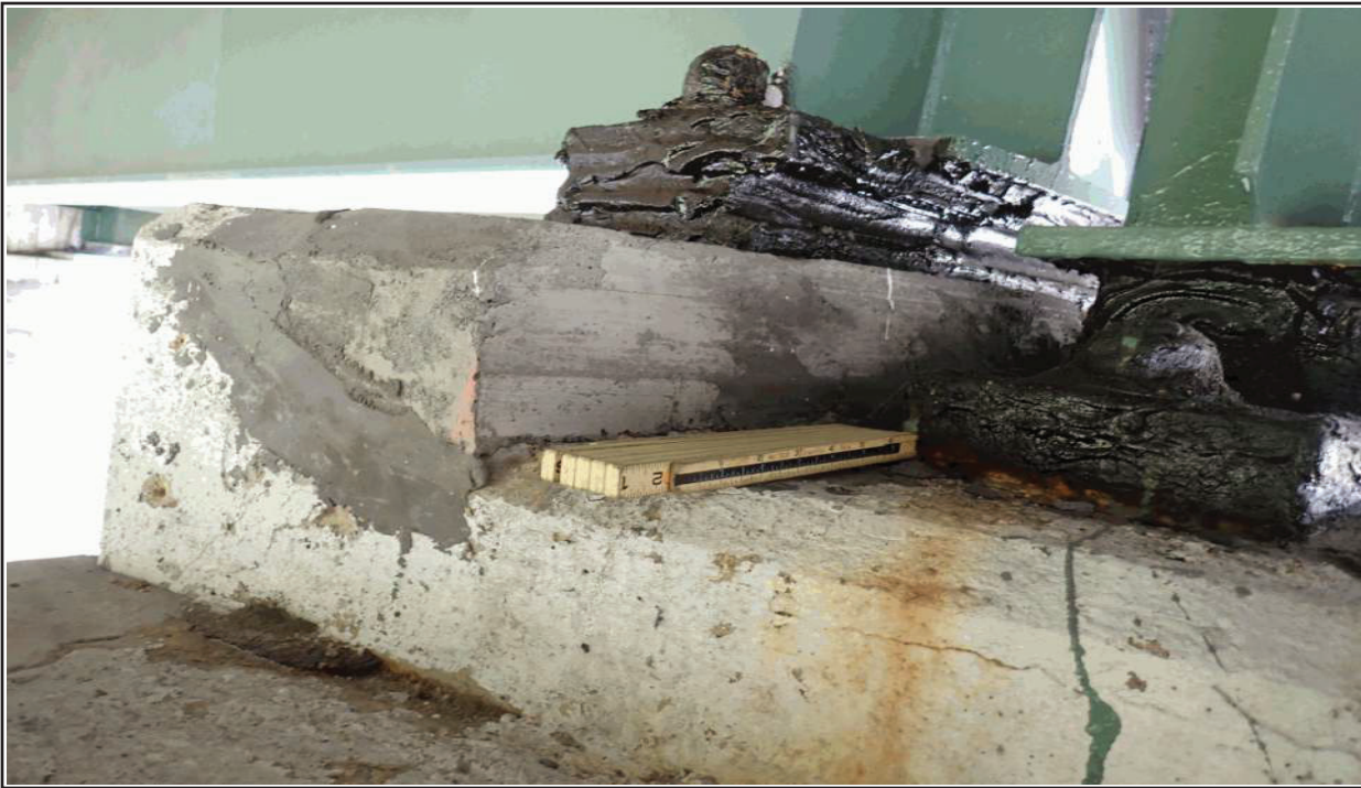
41 PIER 4, SPAN 5, PEDESTAL 4, SOUTH FACE - REPAIRED
