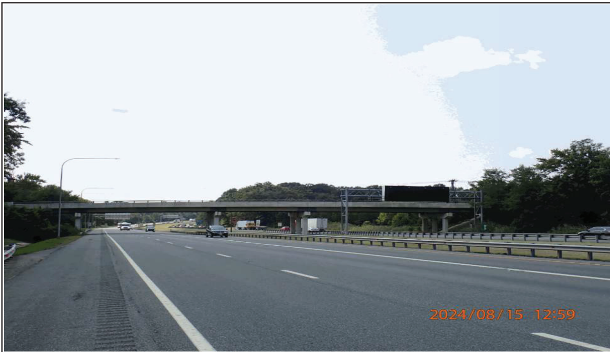
2 EAST ELEVATION, LOOKING WEST
