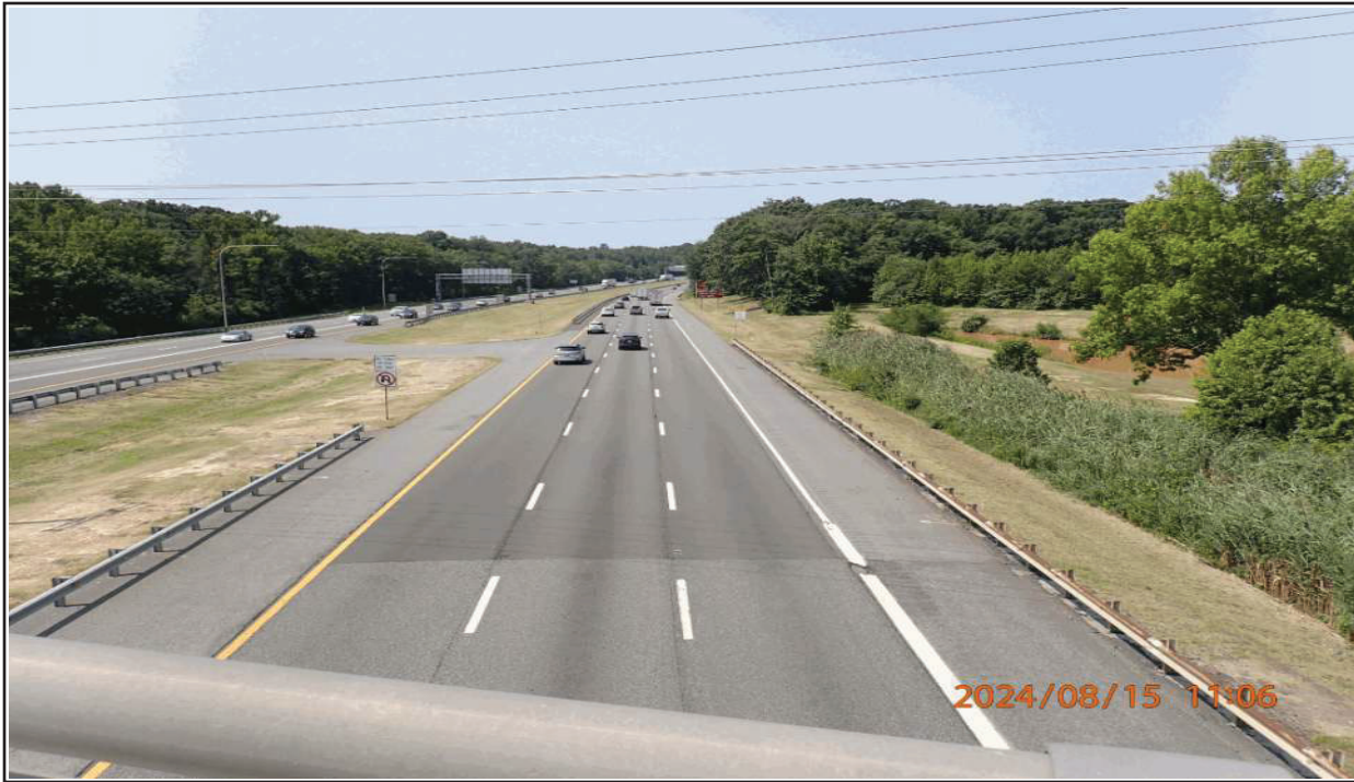
7 UNDER RECORD (SPAN 4 OVER I 95 SB), LOOKING WEST
